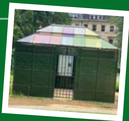
The restored toilets at Sydney Gardens
