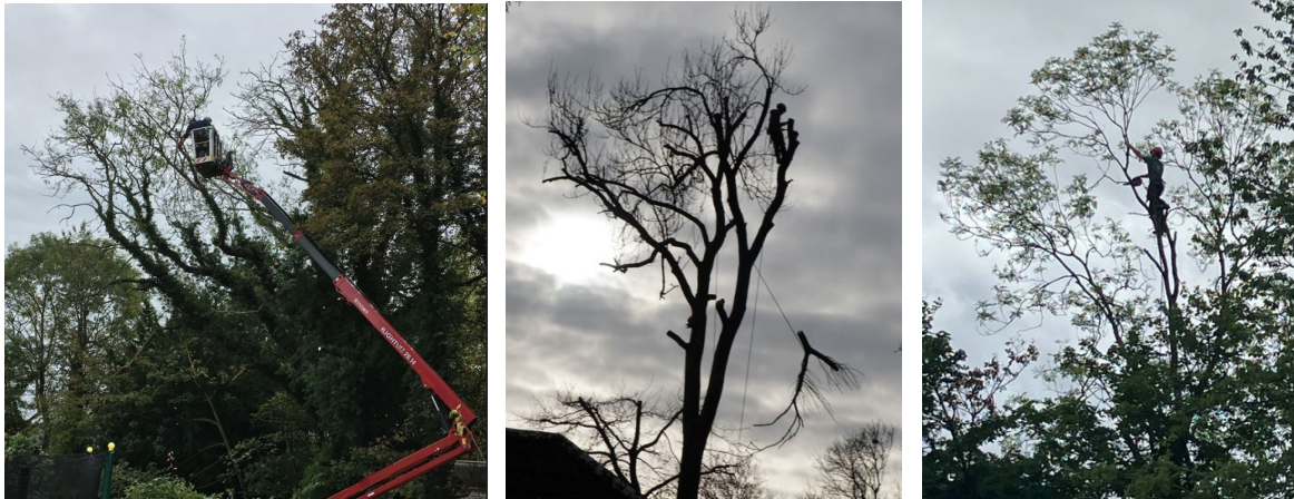
L-R Sectional crown reductions by properties alongside Summer Lane, Combe Down October 2021, December 2022 and August 2025
