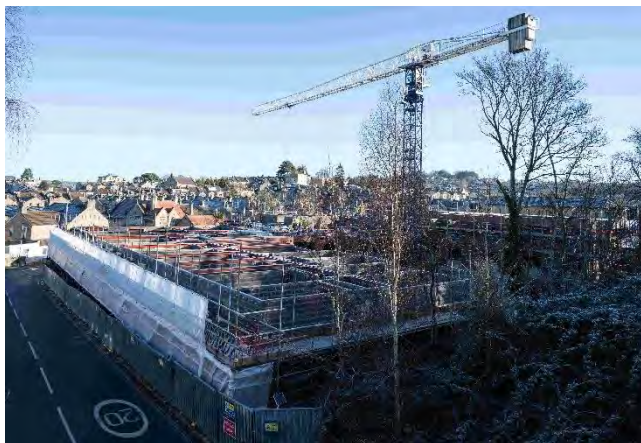
Development site for new care home, January 2025.
