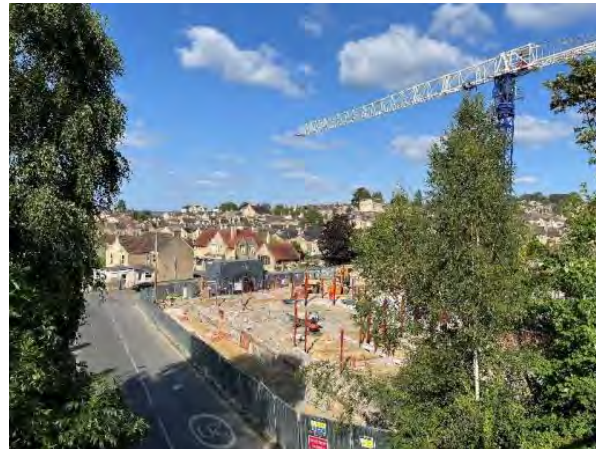
Construction of care home on former ironworks site.
