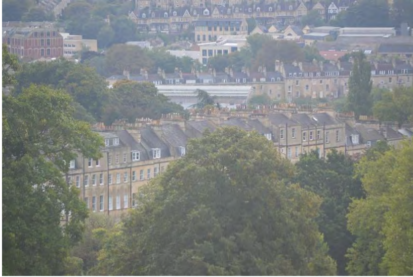
Marlborough Buildings as seen from approach golf course.
