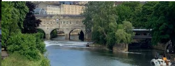
Pulteney Bridge and weir.
