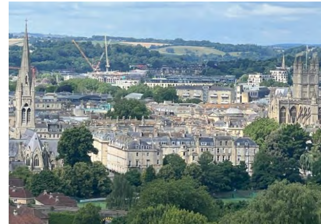
View taken to the west highlighting the new developments of the Western Riverside.
